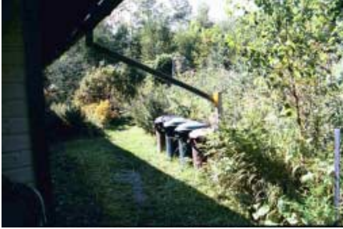
Photo 10 - Hoffman house roof water catchment system and plastic holding containers.
