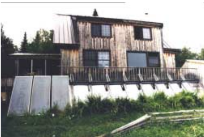
Photo 8 - Abazs house with solar hot water collectors (left foreground) and attached greenhouse (center-right foreground).
