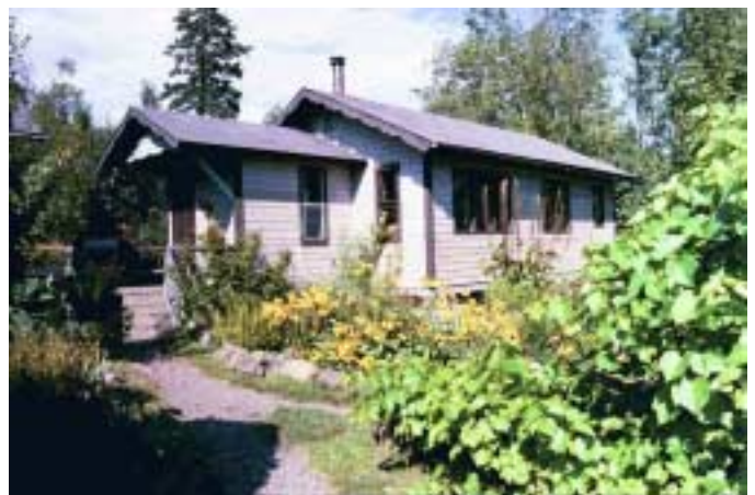
Photo 6 - Hoffman house exterior with unheated entrance annex.
