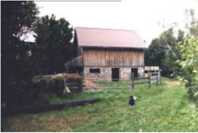
Photo 6- Abazs timber frame barn exterior.
