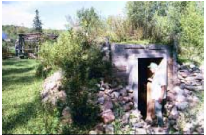
Photo 5- Hoffman root cellar entrance.
